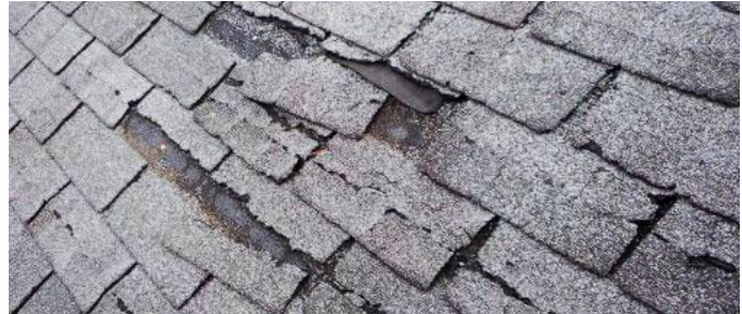
SHINGLE CRACKING & CURLING
