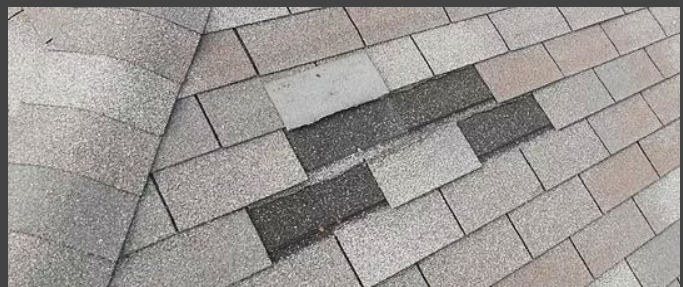
MISSING SHINGLES
