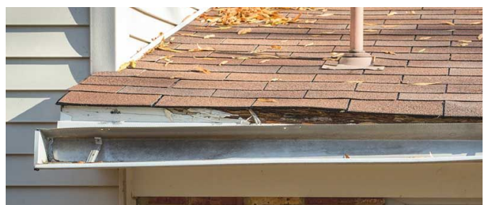
DAMAGED GUTTERS
