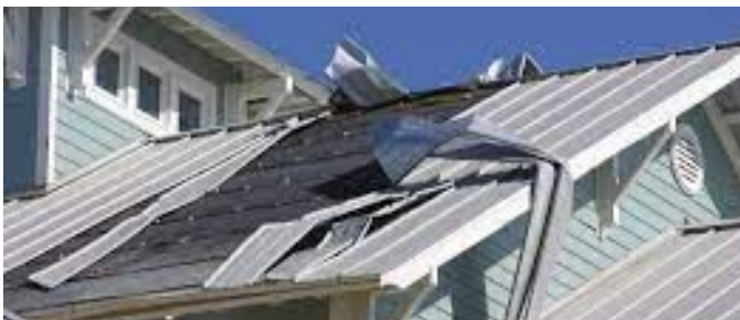
METAL PANEL DAMAGE
