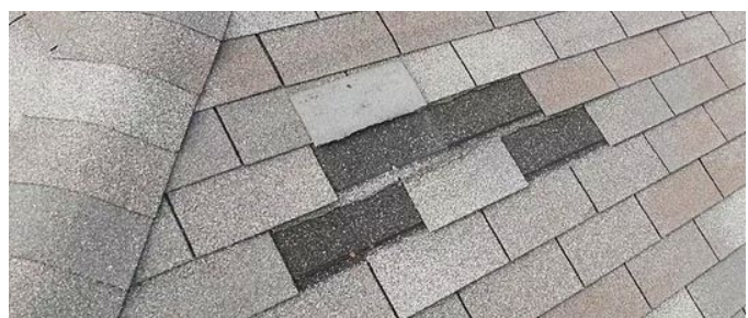
MISSING SHINGLES
