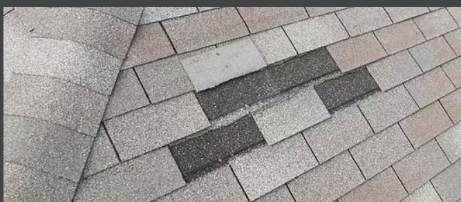
MISSING SHINGLES
